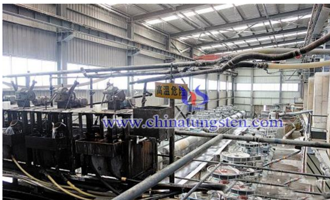
△Flotation Workshop of Tungsten Smelting Plant
